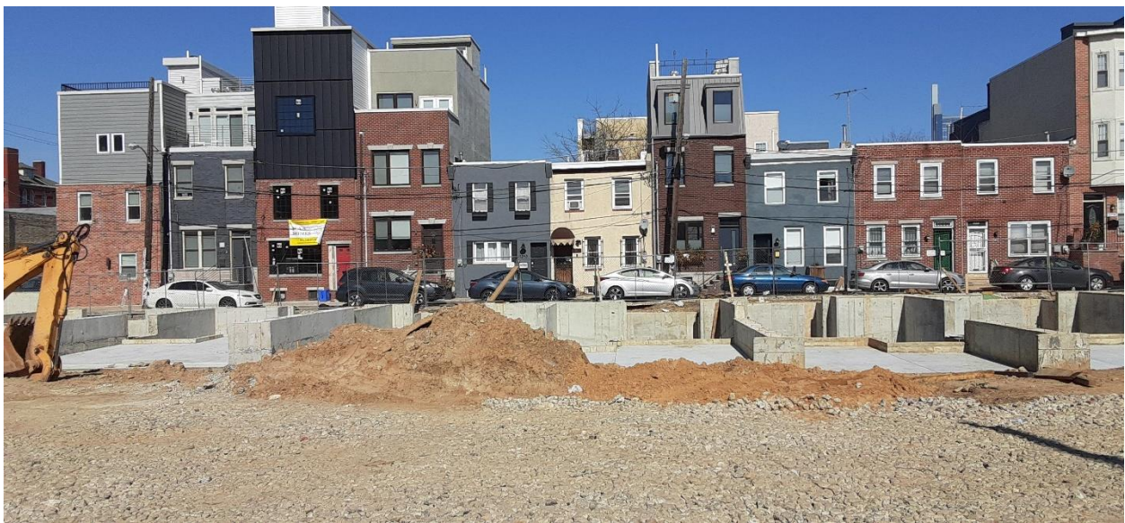
Figure 1, Kimball Street, north of Washington Avenue (Sean O'Rourke)
