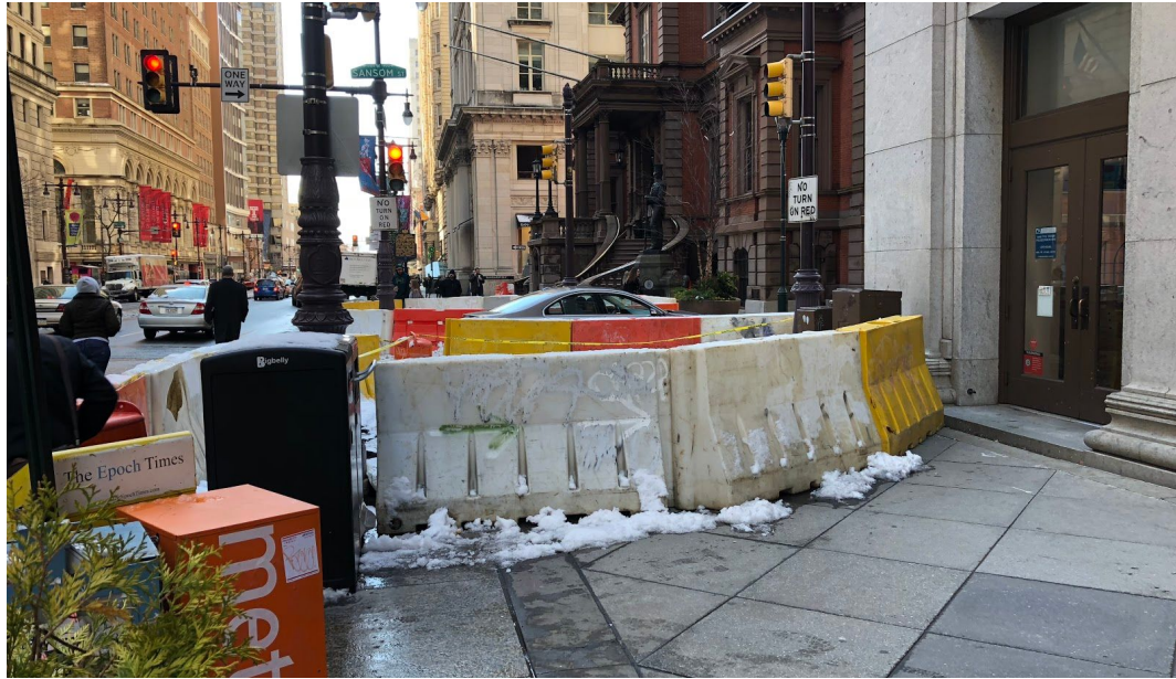
Broad Street sidewalk under construction—totally. (George Claflen photo)
