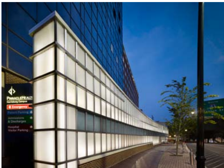
Entrance façade. PinnacleHealth, Harrisburg, PA. Francis Cauffman; Rachel Calemmo, LC LEED® AP. (©2010 Halkin Architectural Photography, LLC)
