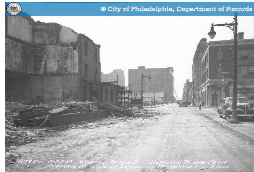
Demolished Building - Vine Street Widening Project
